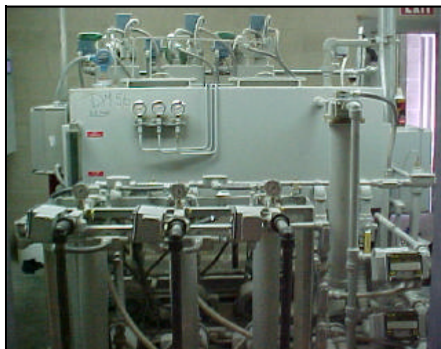
Lubrication system located in lube room
