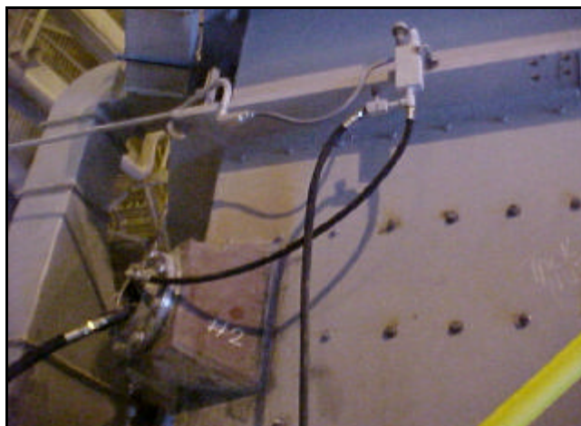
Supply and return oil lines on outside of mill
